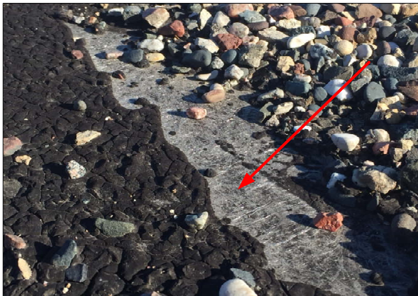
Exposed felts will lead to premature failure of the roof system.
