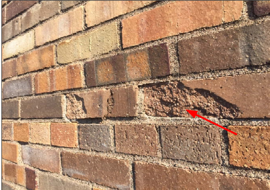
Deteriorated brick/mortar that will need to be addressed during the roof project.
