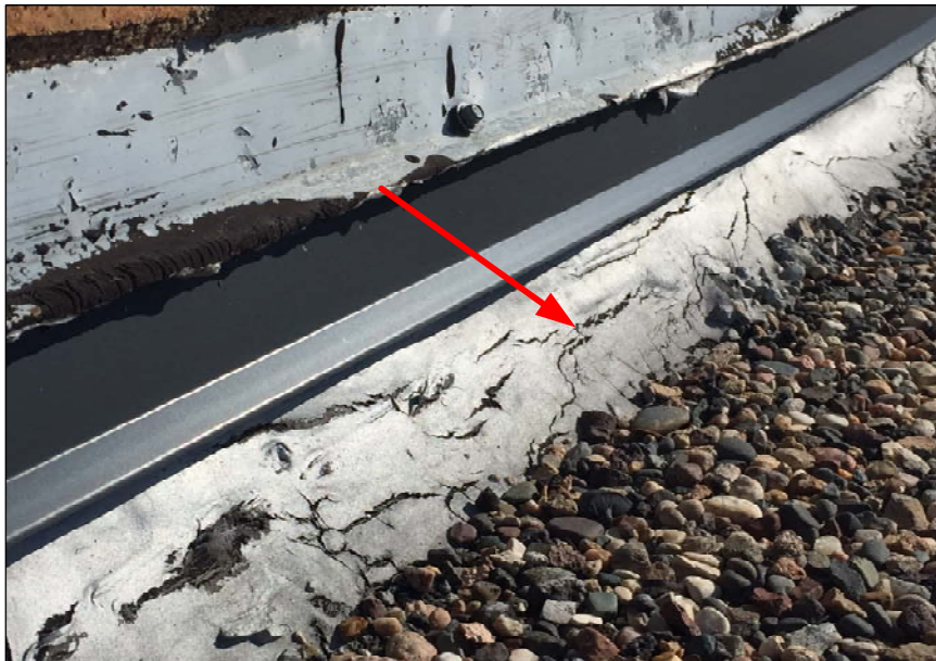
Deteriorated flashings and potential interior leak locations.
