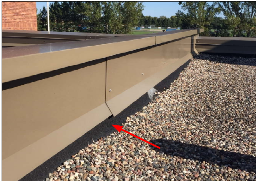
Exposed base flashings that should be coated or covered to avoid further damage.
