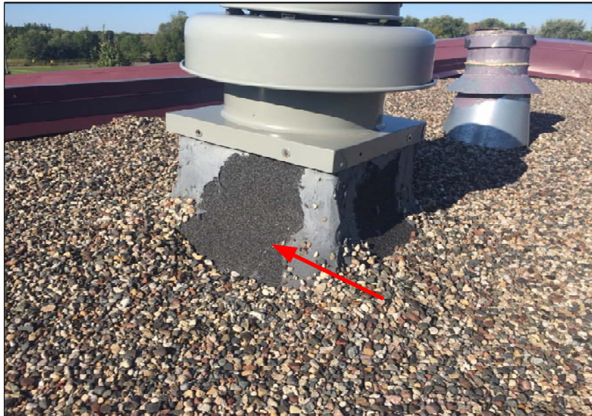
Exposed Flashings
