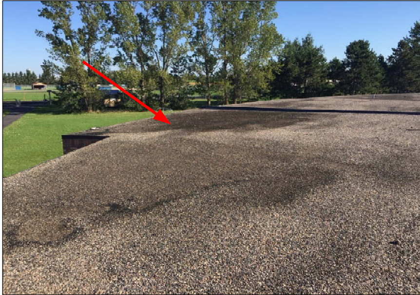
Overview of ponding conditions due to improper slope in the roof surface.
