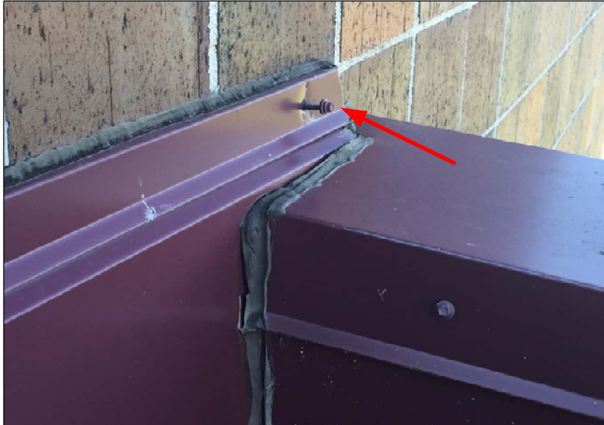
Fastener back out – normal preventative maintenance.
