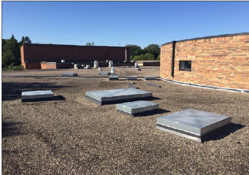
Numerous obsolete curbs need to be removed during the next roof replacement project.
