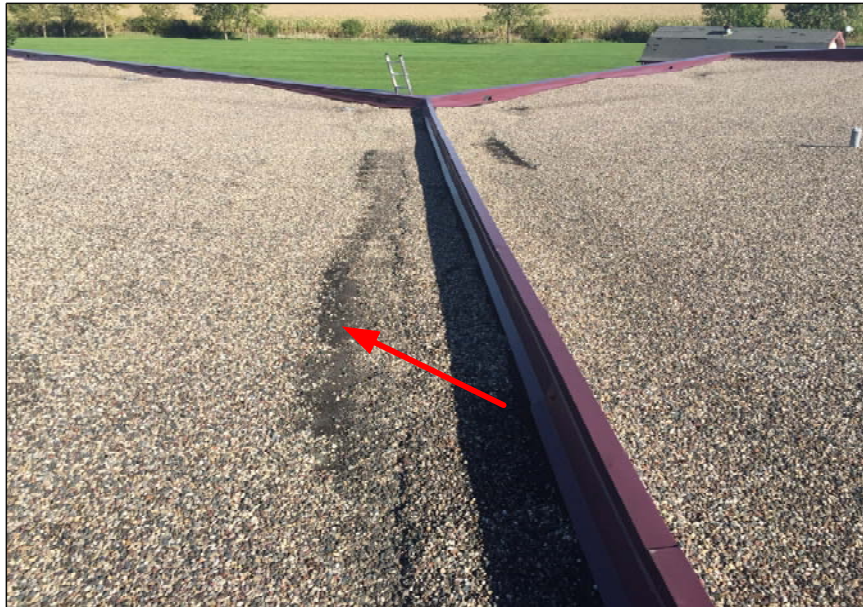
Erosion of the flood and gravel surfacing. Maintenance can be completed to protect these areas of exposed felts.
