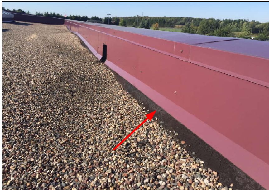
Exposed base flashings need to be coated or covered to minimize future deterioration.
