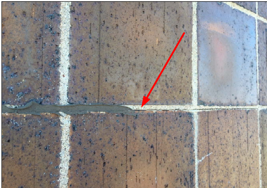
Additional deteriorated mortar leading to leaks.
