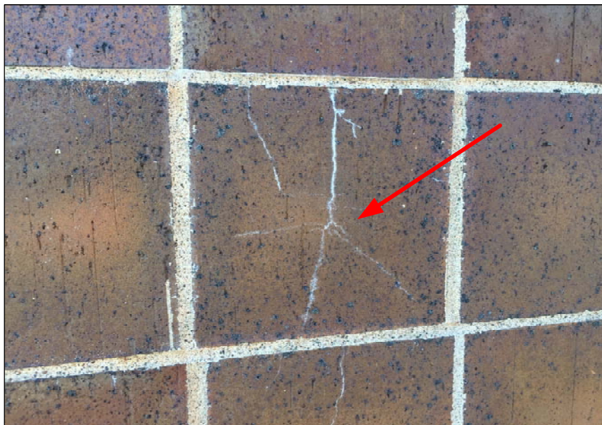
Block deterioration due to infiltration and/or improper drainage.
